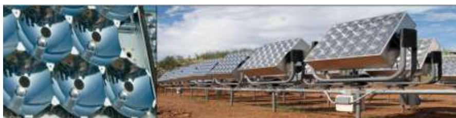
Figure 60. Concentrating Solar PV cell and module
