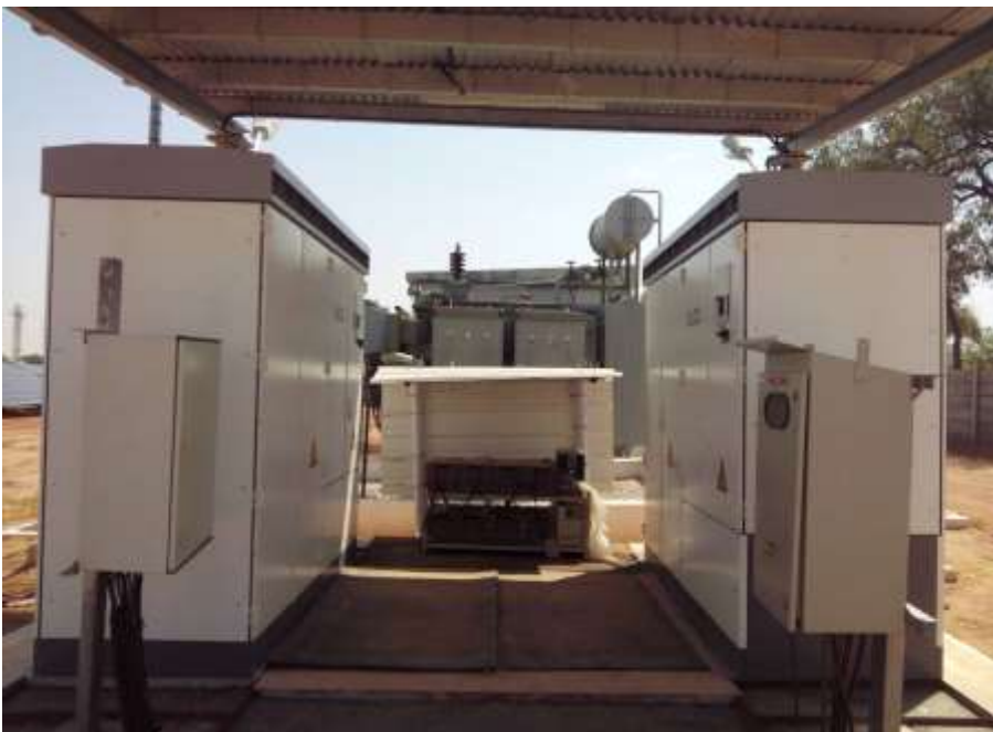
Figure 65. Outdoor Type Inverter Installation
