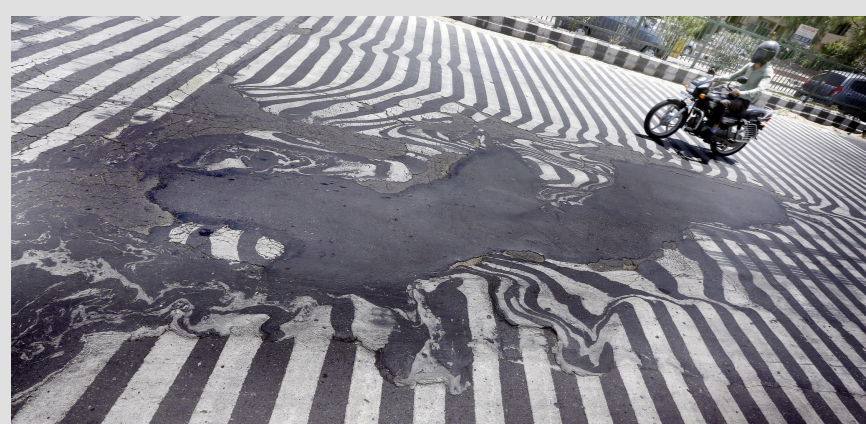
Road melting during a heatwave in India
