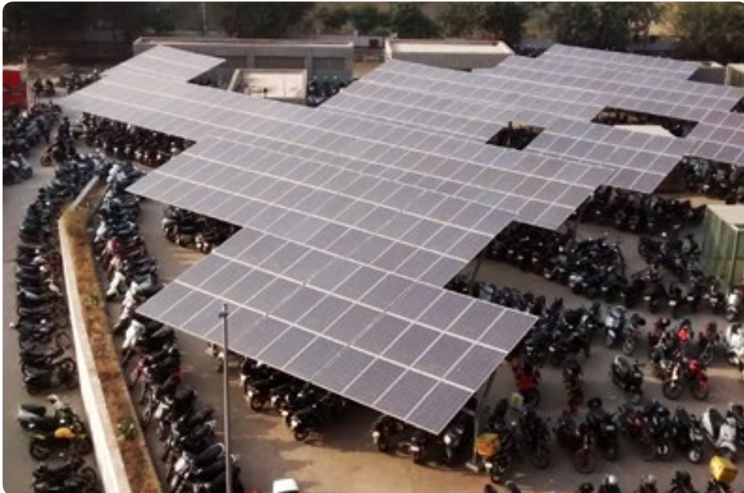
Solar panels are installed in Gurgaon in the state of Haryana
