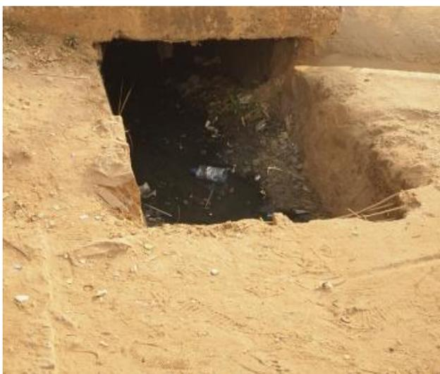
**Figure 3:** Littered drainage channel
