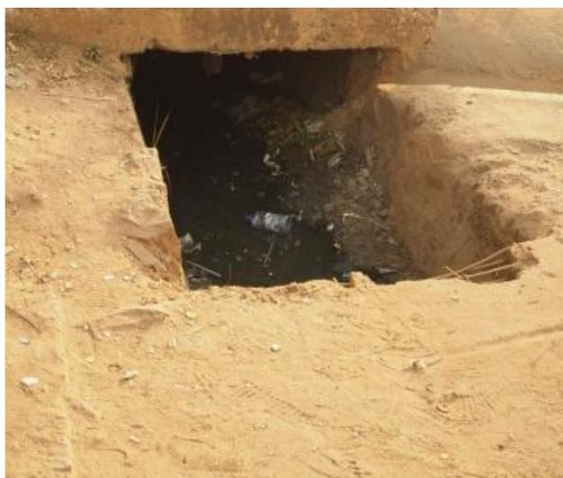
**Figure 3:** Littered drainage channel
