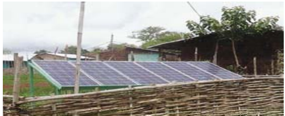
Solar power generation and charging station under construction in a rural community in Ethiopia
