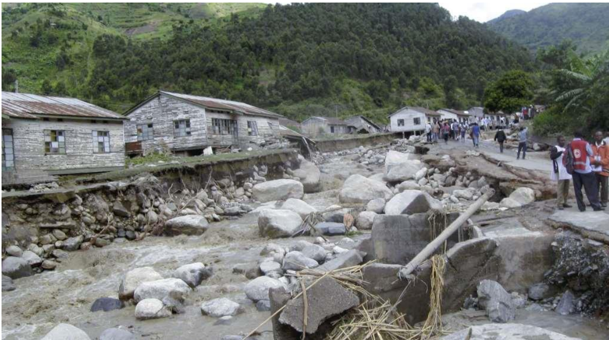
Figure 2: Flood damage to homes and a road in Kasese, Southwestern Uganda
