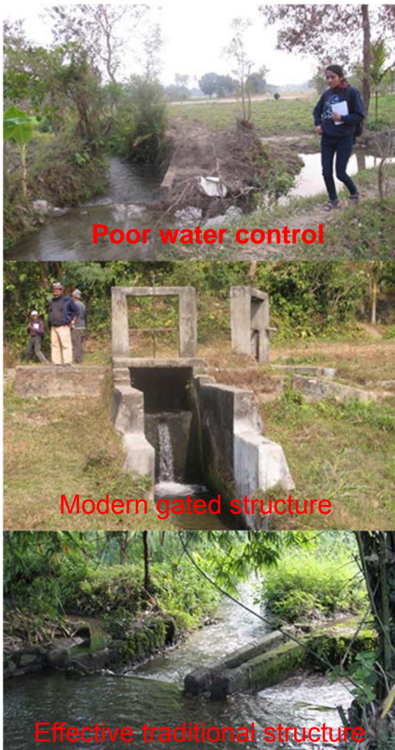
Figure 23: Water Control Structures
