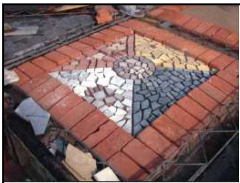
Figure 39 : Funicular shell – various small shell segments can be cast on a grid of beams
