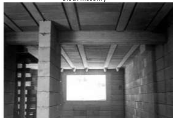
Figure 29 : Low cost housing in Mexico using Concrete Block masonry
