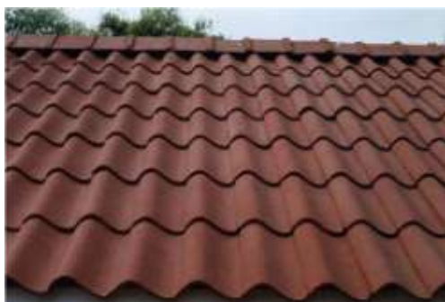
Figure 30 : A roof made of Micro Concrete Roofing Tiles (left) and MCR tile roof in semi-arid Bundelkhand as an alternative for burnt clay country tiles
