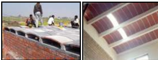
Figure 33 : Precast arch panels in community building (above), view of the ceiling
