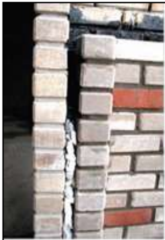
Figure 40: Cavity Wall with Waste Thermocol Infill
