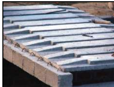
Figure 31: Plank and Joist Roofing
