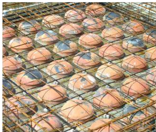
Figure 37 : Ceiling of earthen pot filler slab, Auroville (above) and Reinforcement details & earthen pot positions (below)
