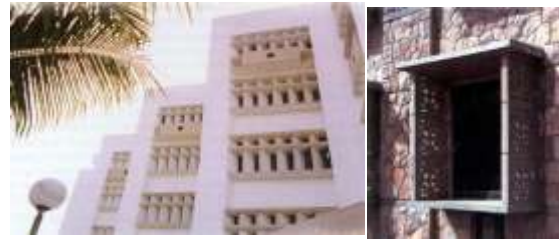
Source: A. B. Lall Architects; Best Renewable Energy Development Agency (WBREDA).
