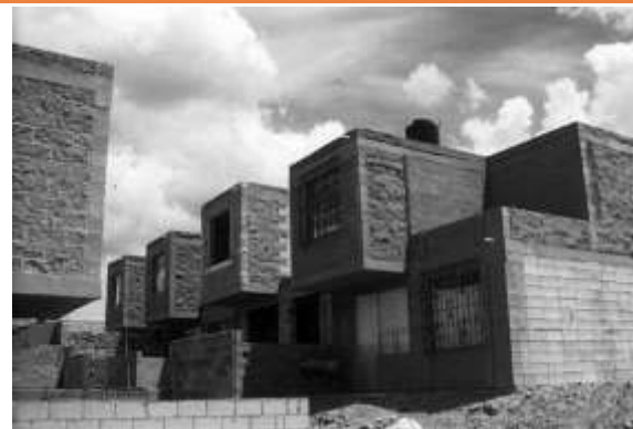
Figure 29 : Low cost housing in Mexico using Concrete Block masonry
