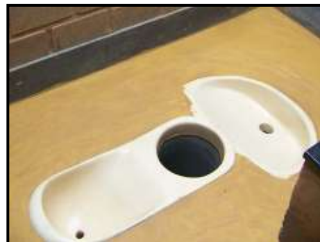
Figure 41: Ecosan Toilet on a Raised Platform with Waste Storage below (above), Ecosan Pan for Waste Separation (below)
