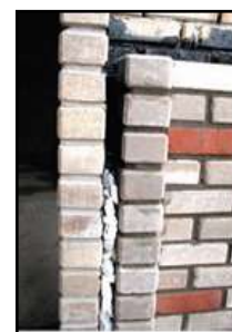
Figure 27: Cavity wall with waste thermocol infill
