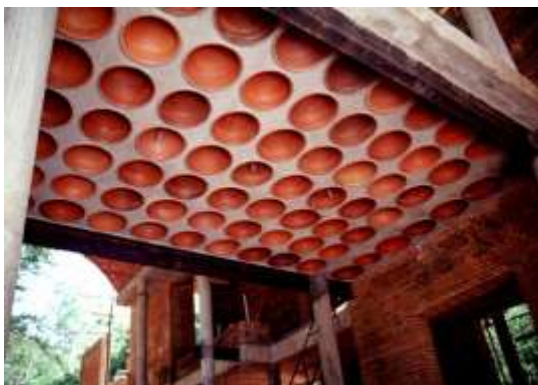
Figure 37 : Ceiling of earthen pot filler slab, Auroville (above) and Reinforcement details & earthen pot positions (below)
