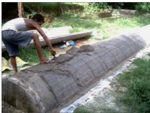
Figure 36 : Manual Production of Ferrocement Channel (above) and Office Building in TARA Gram, Orchha (below)
