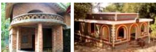
Figure 26 : Cyclone resistant community building in Rat-trap bond by Orissa Development Technocrat's Forum, Right – House in Kerala in Rat-trap bond
