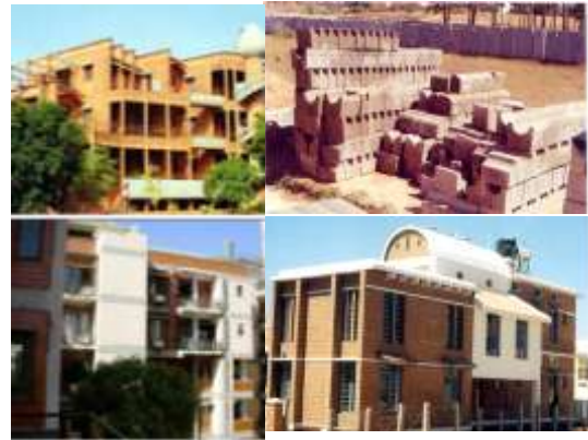
Figure 24 : Stabilized Compressed Earth Blocks – Projects. (Clockwise from top left) – Multi-storeyed apartments in Auroville, Tamil Nadu, CEB block types, Residential building by IISc. Bangalore, Zero energy residential development in Bangalore by BCIL
