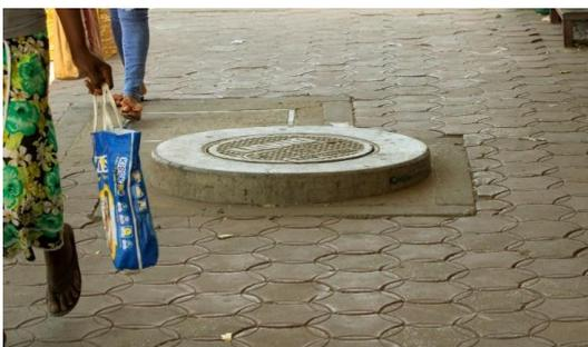
Internet, electricity, and telephone service providers had installed manholes that rose above the pathways obstructing movement especially for PWDs particularly in Digo Road.
