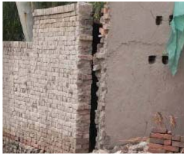
Effects of poor bonding at corners - Jatoi Punjab
