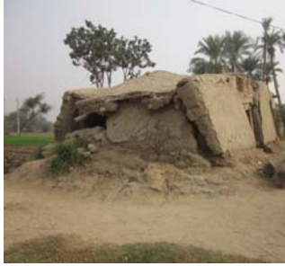
Damaged mud walls due to foundation damage, Punjab
