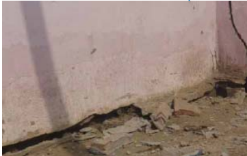
Erosion at base of wall - Punjab
