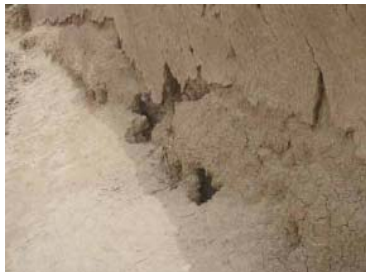
Rainwater erosion to the base of a mud wall - Balochistan
