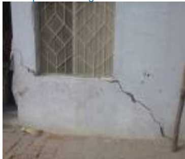
Earthquake damage to rural home
