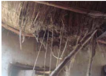
Ponding of rainwater on a flat roof leading to collapse - Balochistan
