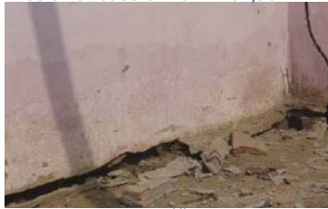
Erosion at base of wall - Punjab
