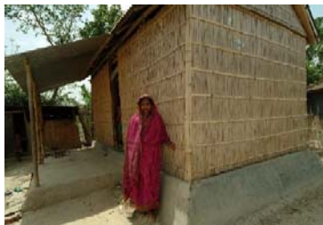
Solid Frame House with Bamboo Walls
