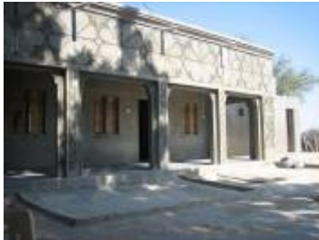
Example drainage off roof eaves, down-pipe missing, Thar Desert, Sindh
