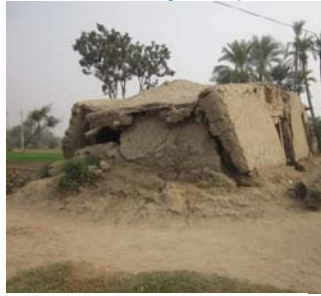
Damaged mud walls due to foundation damage, Punjab
