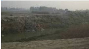
Example of damaged flood bunds post 2010 floods
