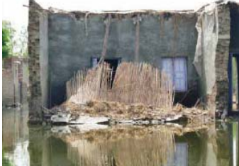
Overturned wall due to foundation settlement - Muzaffargh, Punjab
