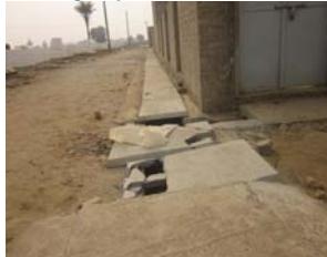
Example damaged closed drainage system
