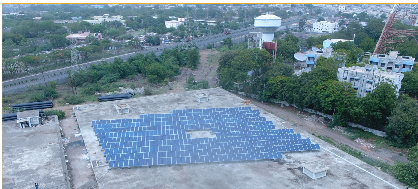
A 145 kWp grid-connected solar PV system at the Aji water treatment plant.
