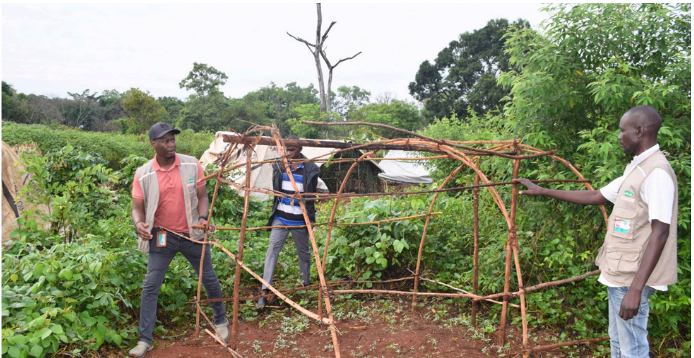
YEDA team constructs emergency structures in Western Equatoria. Photo credits: YEDA
