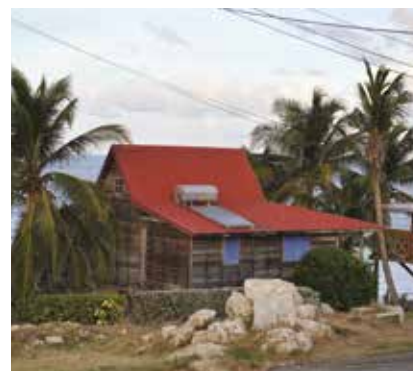
Image: Kate Shifman | Barbados, Solar Water Heater
