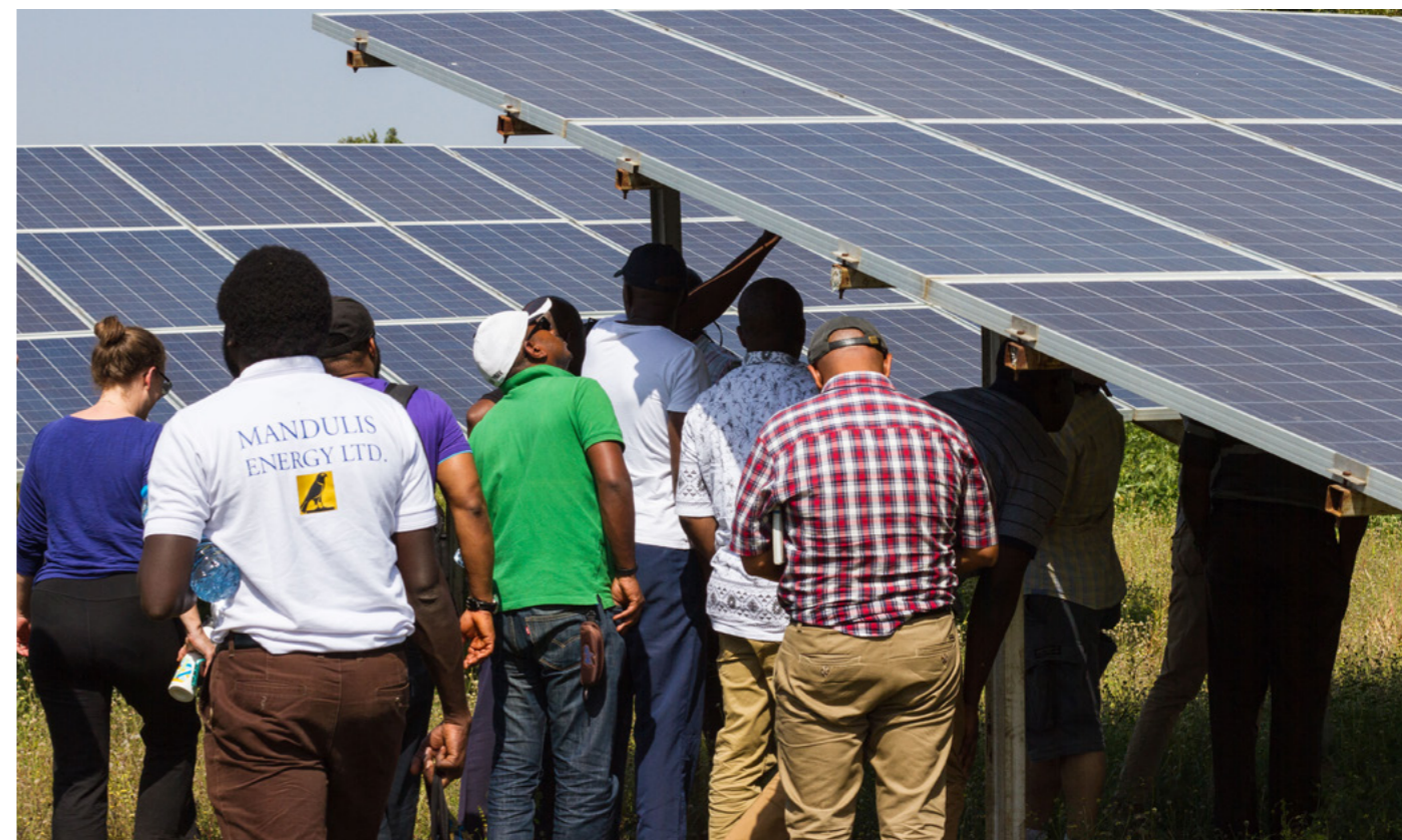
Image: © LEDES GP | Study tour of solar-powered rural electric grid, Nigeria.
