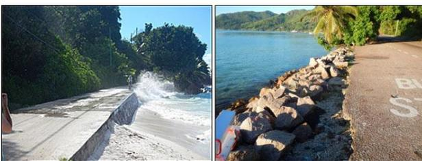
Figure2: Vulnerable coastal infrastructure and rock armouring interventions (Photo credit: van Prosdij and Baker, 2015)
