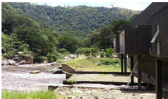
River Mpanga power station
