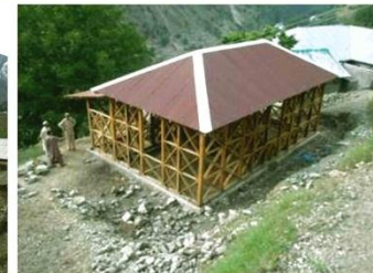
3. Tin roof cladding fastened over roof structure
