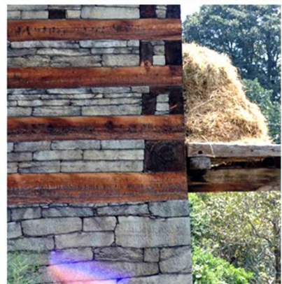
Elevation and corner views of timber reinforced stone masonry
