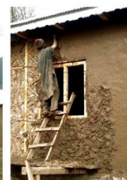
5. Mud plastering of walls
