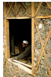
4. Dhajji walls constructed. Timber framework and cross bracing are filled in with stone
