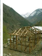
2. Timber framework of walls and roof erected
