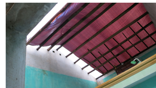
Bottom: The roof of Ms. Nguyen Thi Luong was blown off due to an insecure connection between the roof covers and roof structure.
