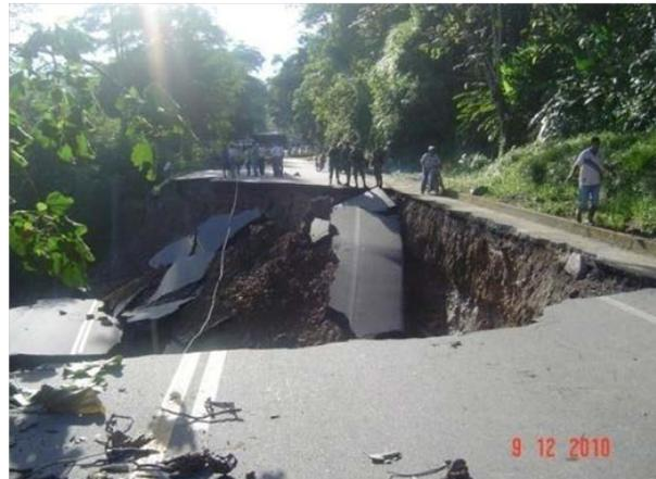
Figure 16: Caved-in roadway due to erosion between Bucaramanga and Barrancabermeja. Source: Ministry of Transport, 2012a.
