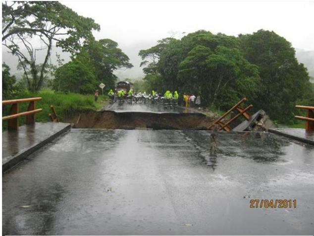
Figure 7: Collapse of “El Mochilero” bridge near San Jose del Fragua by scour on the abutments. Source: Ministry of Transport, 2012a.
