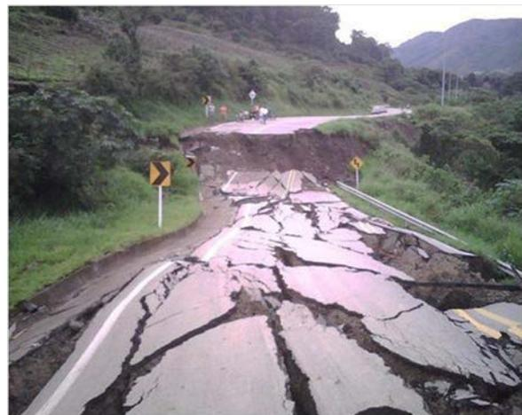
Figure 1: Road damage from erosion and scour between Cucuta and Pamplona. Source: Ministry of Transport, 2012a.
