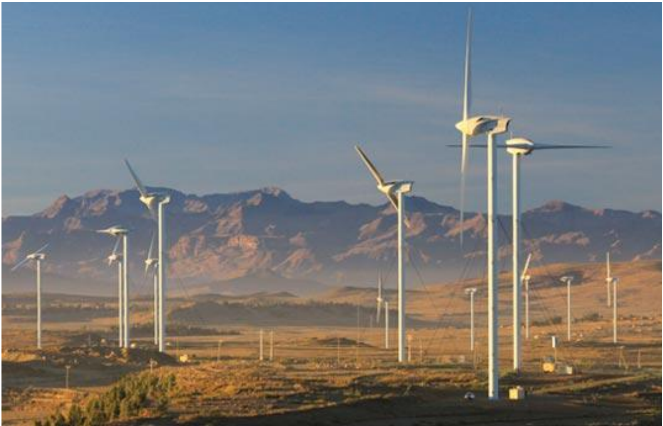
The Ashegoda Wind Farm, which at 290 Million USD is the largest investment in the wind energy in Sub-Saharan Africa. The wind farm is expected to generate 120MW of electricity, easing Ethiopia's dependence on hydropower.
